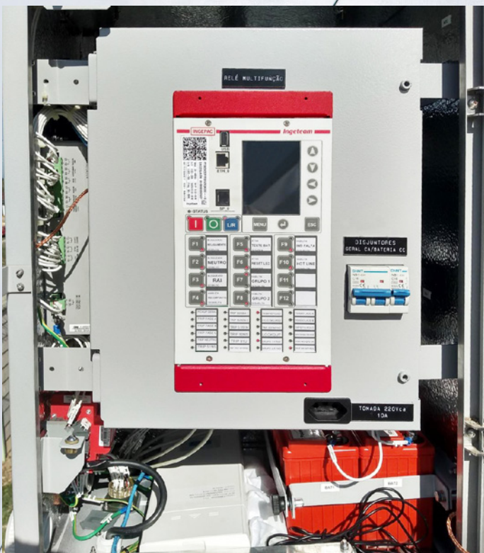
INGEPAC™ DA PT installed in a cabinet
